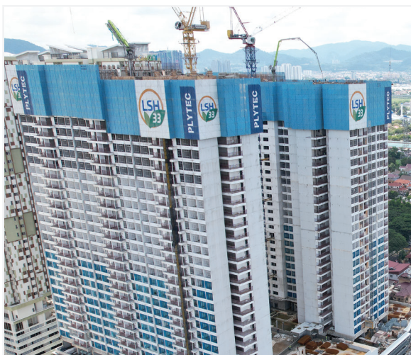
(Steel Frame & Chain Hoist Lifting System)
