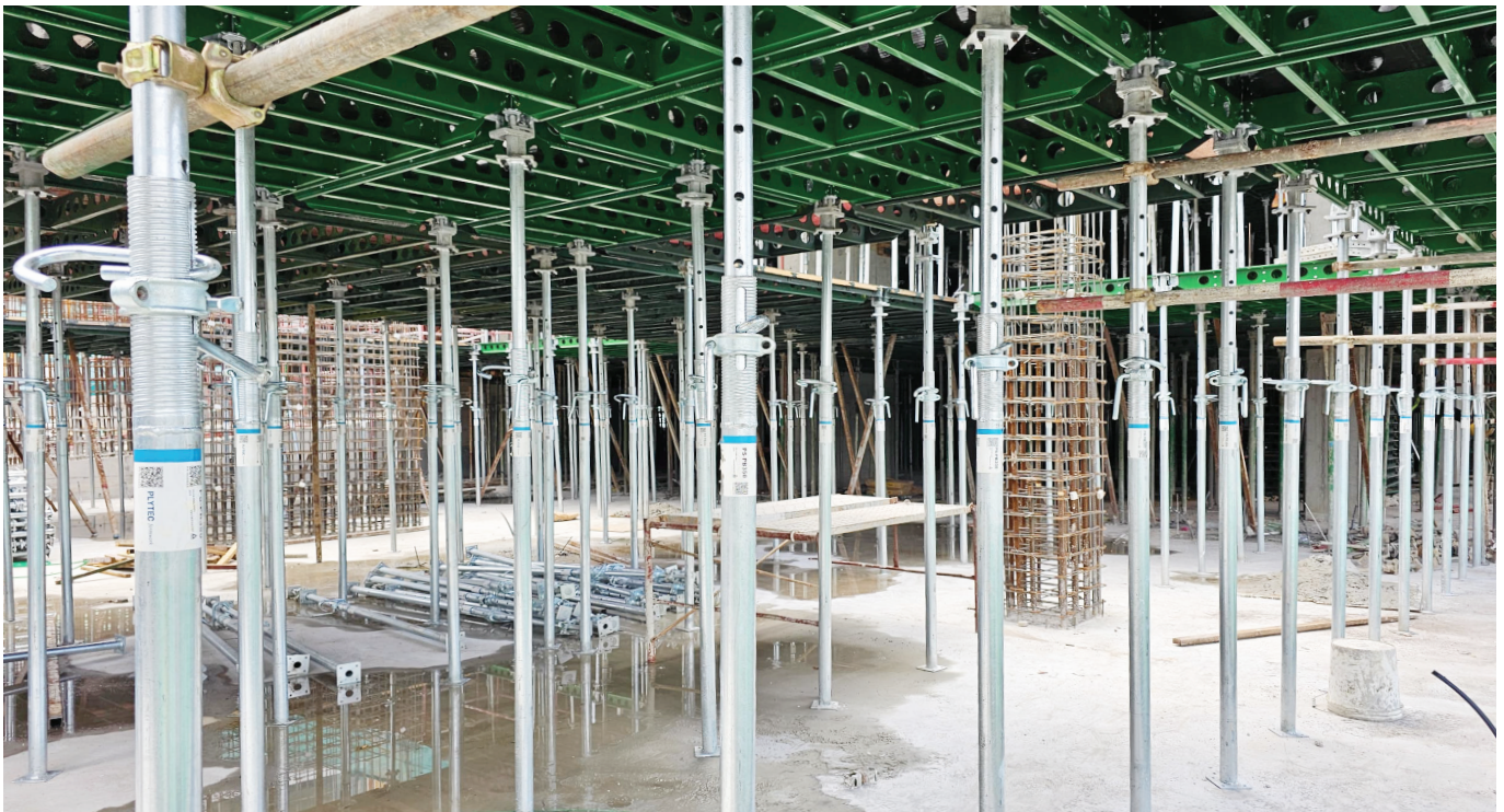
Falswork & Formwork
